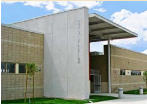
Curtis Middle School, New Campus
