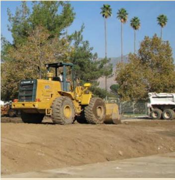
Sitework is underway with earthwork and demolition of existing concrete parking slab.
