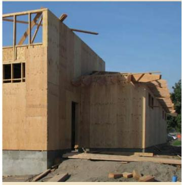
Rough carpentry work continues with plywood siding and roof trusses enclosing the structure.
