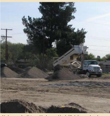
Underground utilities stubbed out and back filled; formwork and concrete for foundation pad are next.
