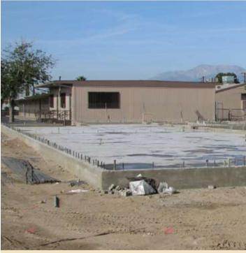
Concrete foundation pad poured, framing to start.
