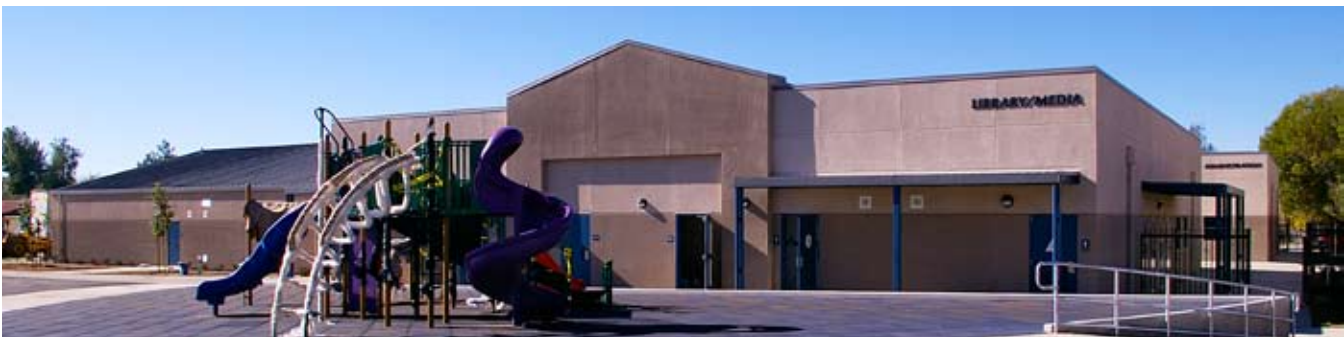
Rodriguez PREP Academy, playground and Library/Media Building
