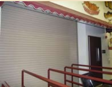
○ San Andreas High School, Kitchen Upgrade
