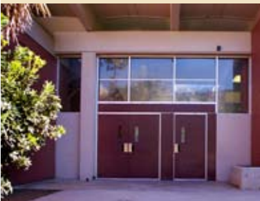
○ Shandin Hills Middle School, ADA-Compliant Door and Entryway
