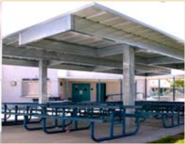
○ Palm Ave Elementary School, Lunch Shelter
